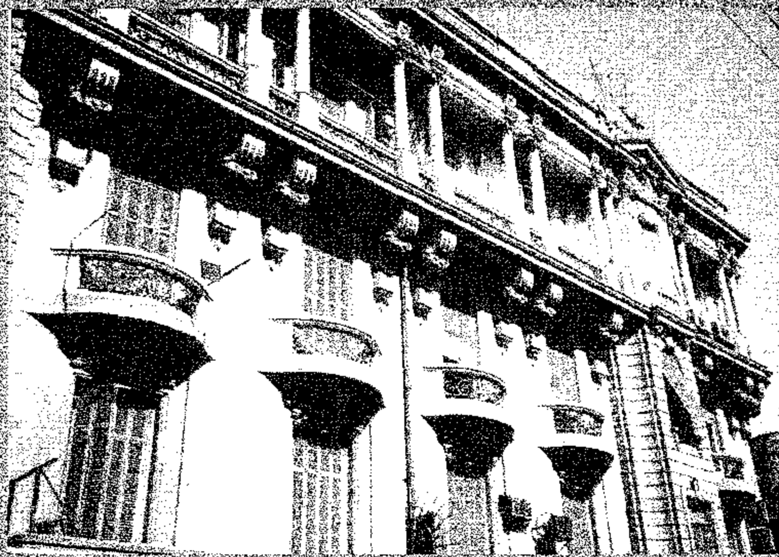
1 Suq El-Tawfikia St. Details of elevation overlooking Suq El-Tawfikia St.
